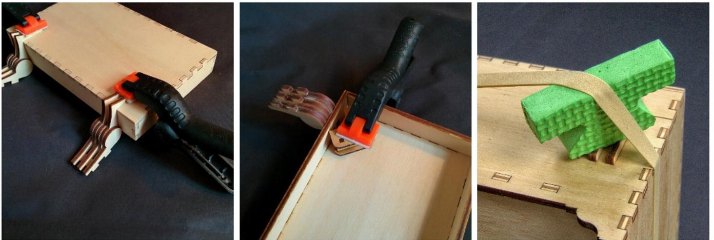
Test fit the lower part of the hinge and notice where it touches the box. This is where the glue will be applied. Glue both hinges at the same time. Apply glue where the hinge will touch the box, including inside the cutout edges, and fit the hinges to the back of the box. Put a rubber band around the box, over the hinges. Use a spacer to send some of the band's pressure so it presses the hinge against the box. Set aside for the glue to dry.
